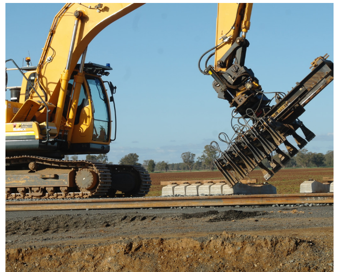
Rail sleepers laid by specialised machinery
