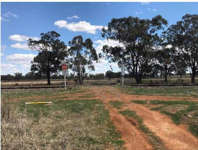
Figure 1: Dows Lane Level Crossing September 2018
