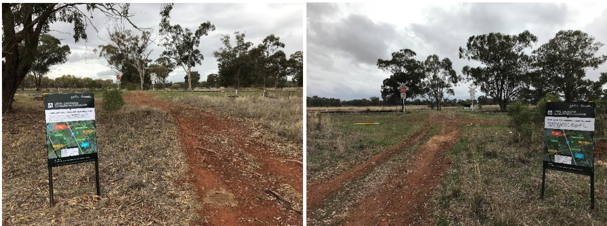
Figure 7: Signage installed at Dows Lane level crossing
