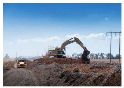
Removal of the rail and formation (the foundation of the track)
