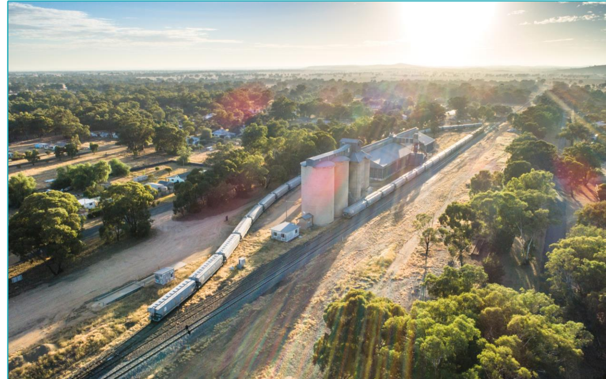
Existing rail infrastructure in Stockinbingal
