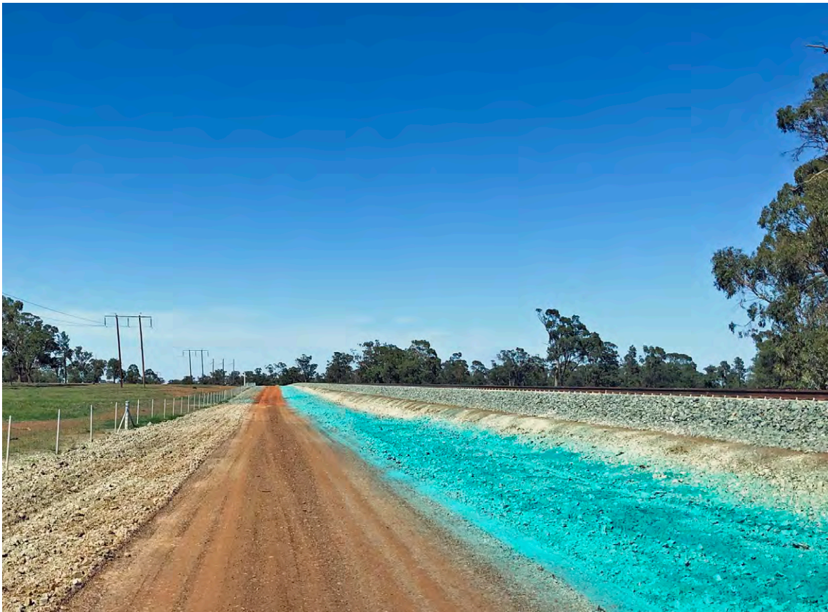
Hydromulch application near Goonumbla.
