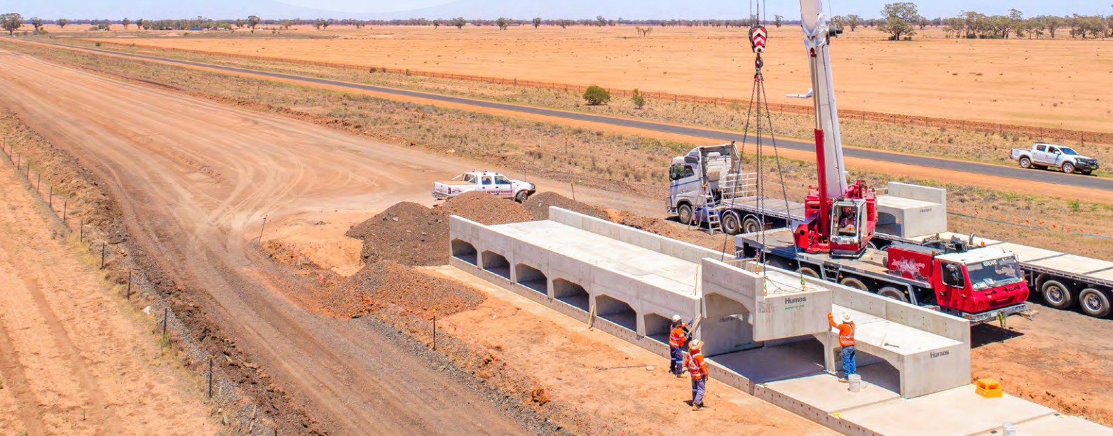
Carbon neutral culverts being installed on the Parkes to Narromine project.
