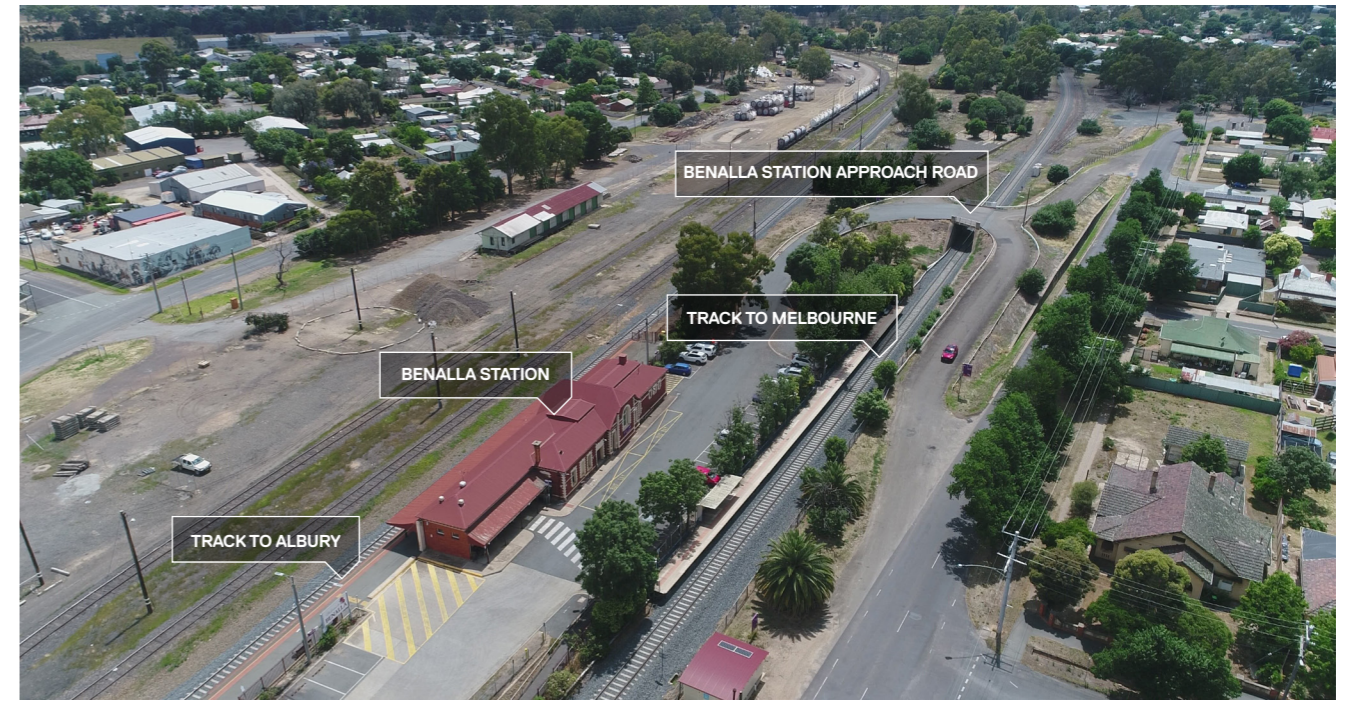
Aerial view of Benalla Station and Benalla Station Approach Road
