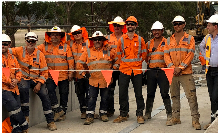
Cutting the ribbon on the last bridge deck conversion near Glenrowan. 82 timber top bridges have been replaced with new ballasted concrete deck bridges resulting in a smoother ride.
