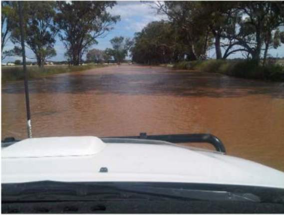
Local flooding Tomingley Road 2012
