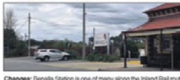
Changes: Benalla Station is one of many along the inland rail route that will require alterations to accommodate double-stacked trains.
