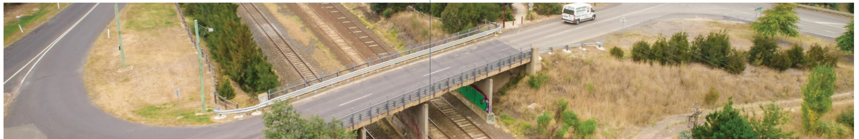
Existing Broadford-Wandong Road bridge in Broadford.
