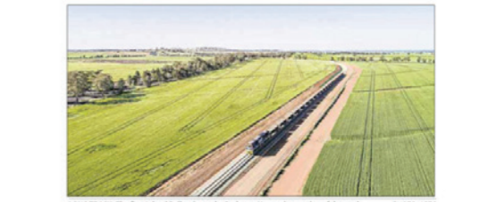
LONG TRACK: The first Inland Rail train on the Parkes to Narran section of the track. PHOTO: ARTC
