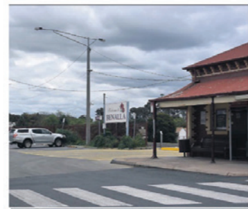
In focus: Benalla Station is one of many along the Inland Rail route that will require alterations to accommodate double-stacked trains.
