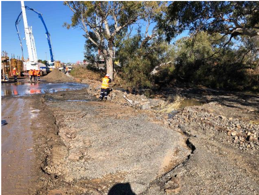
Plate 23 – Gurley Creek Bridge erosion to pad following rain event.
