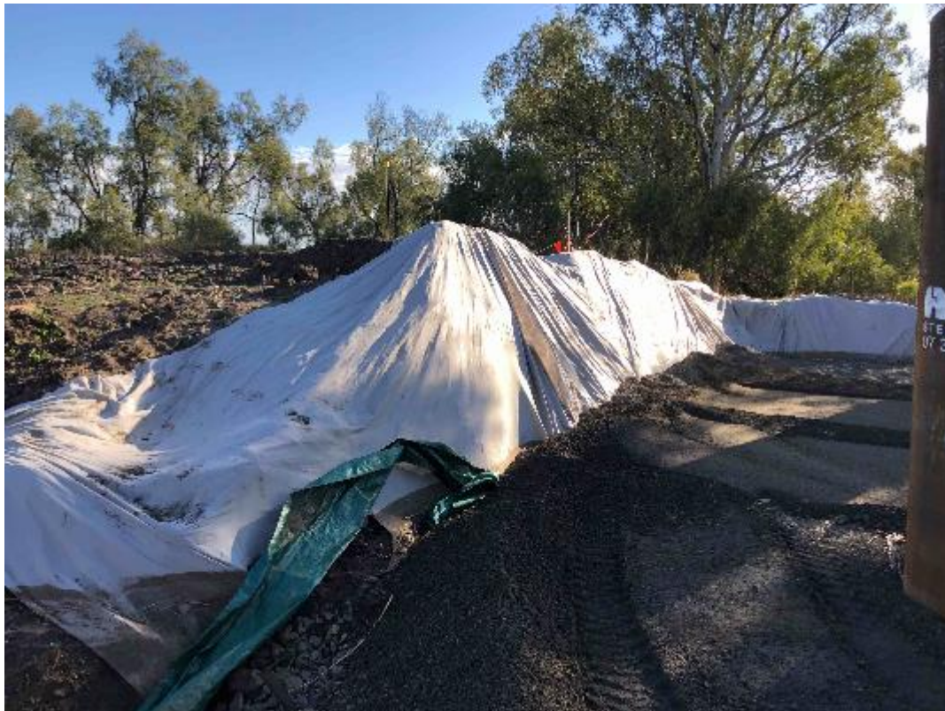
Plate 9 – Yallaroi stockpiles covered with geofabric
