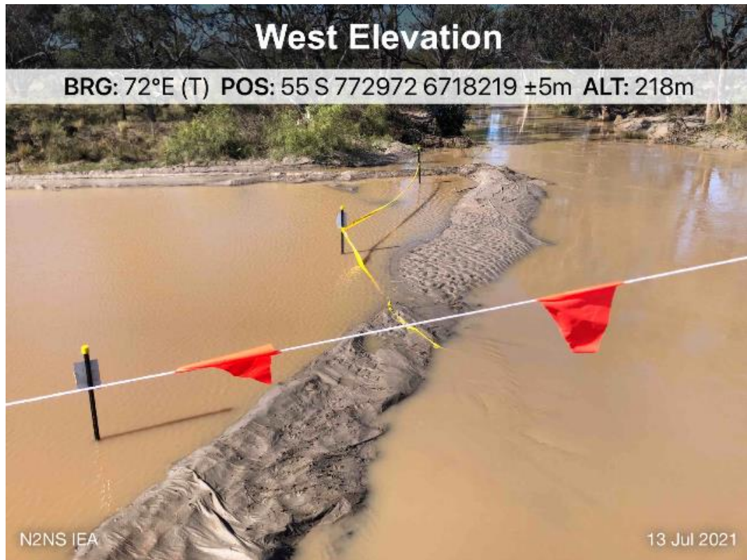
Plate 31 – Gurley tributary sediment controls following rain event.
