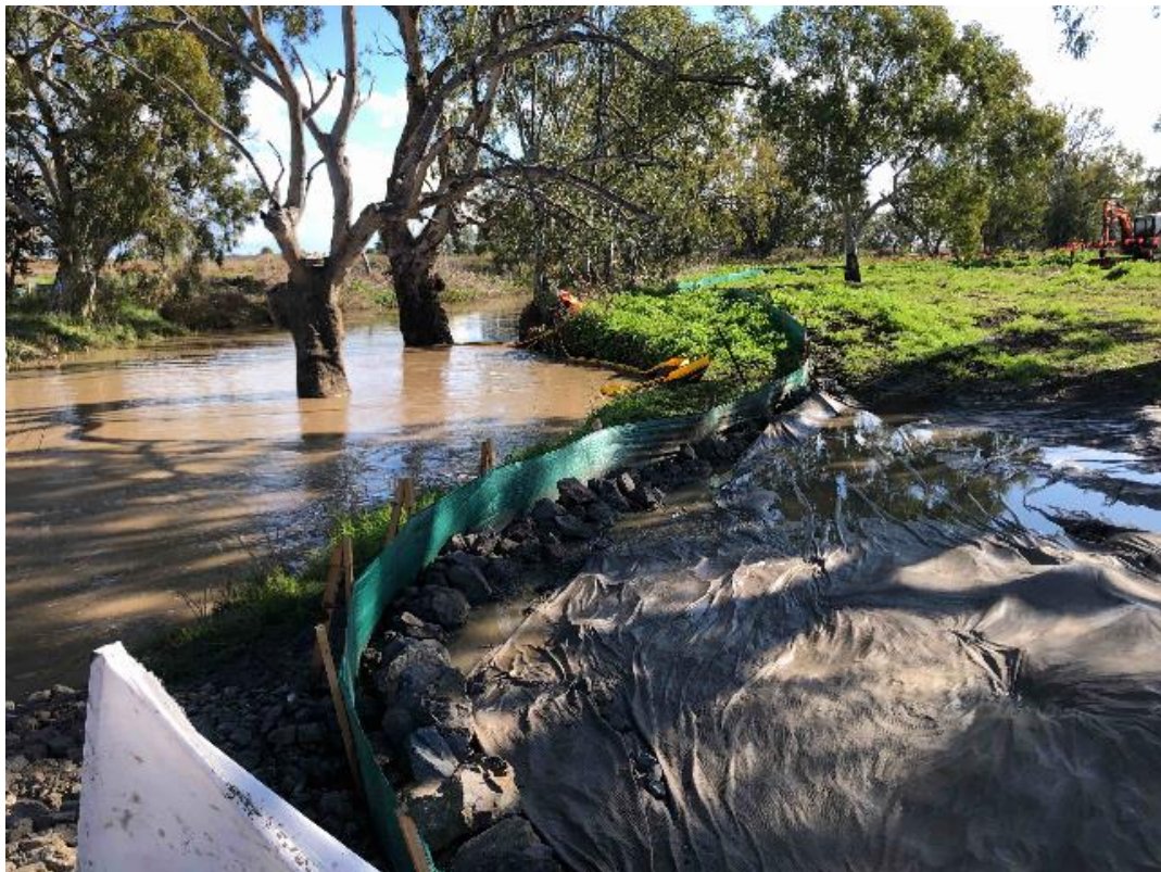
Plate 6 – Yallaroi Creek sediment control repairs during site inspection
