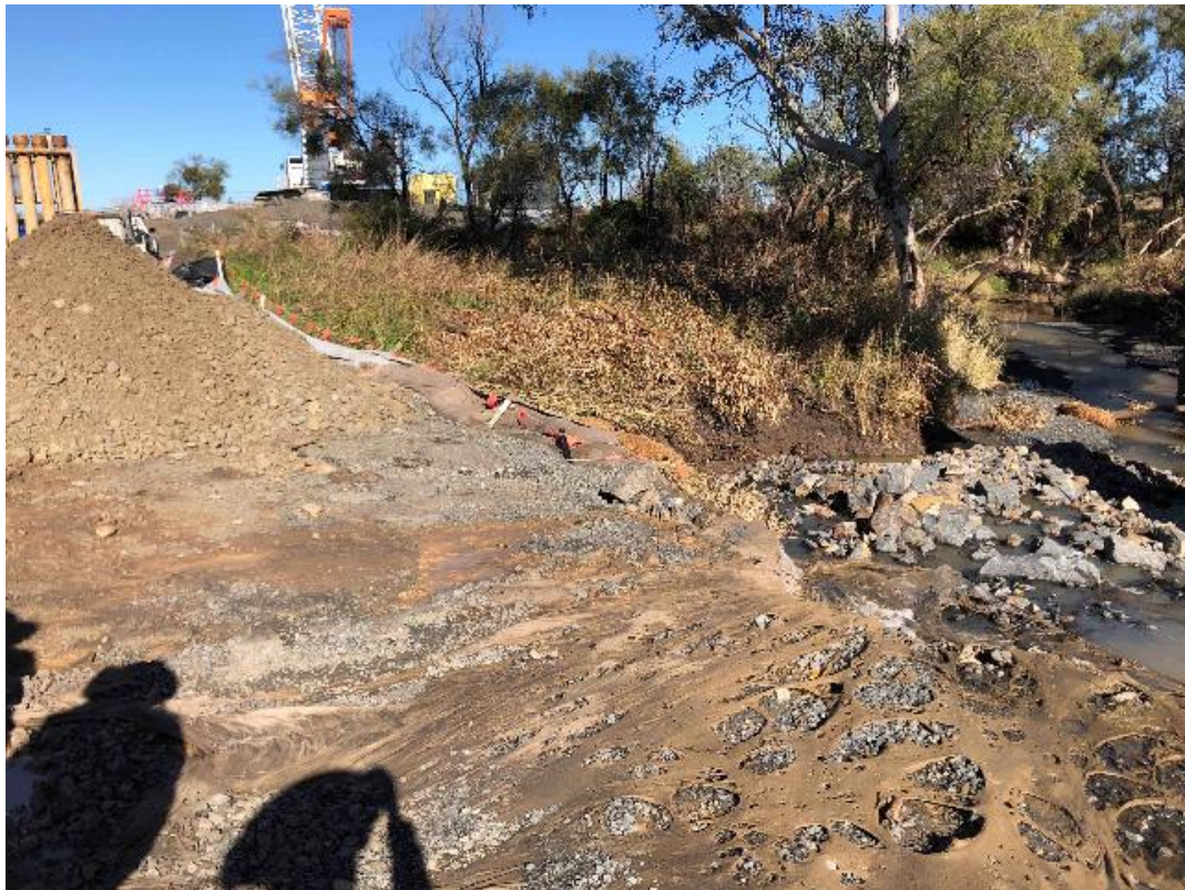
Plate 21 – Gurley Creek Bridge erosion to pad following rain event.
