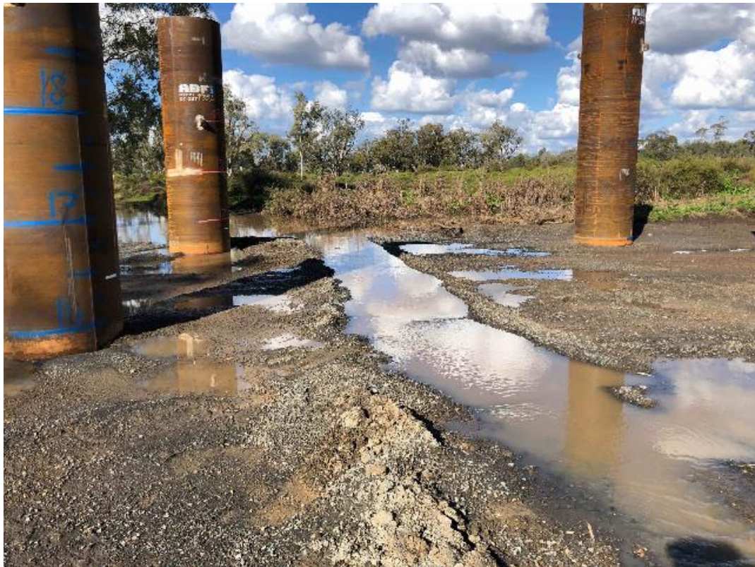
Plate 7 – Yallaroi Creek erosion of pad following rain event
