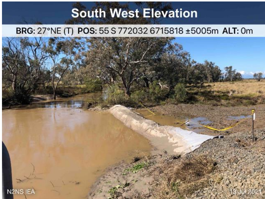
Plate 29 – Gurley tributary sediment controls following rain event.
