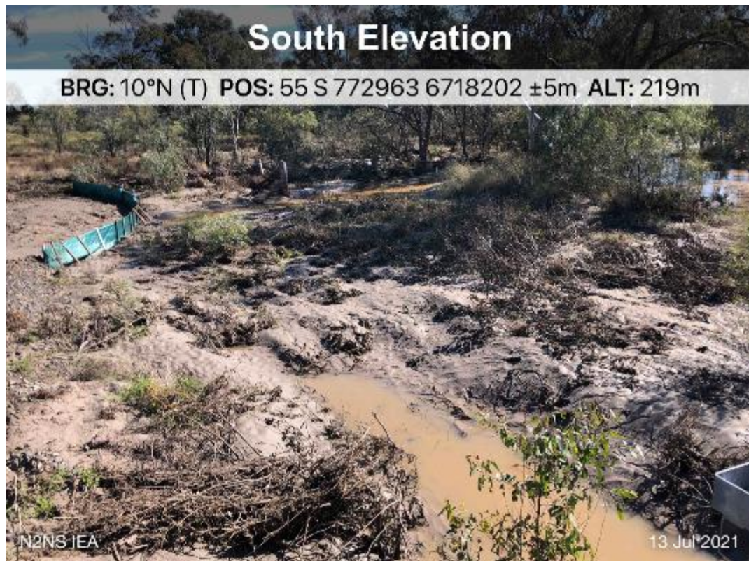
Plate 30 – Gurley tributary sediment controls following rain event.
