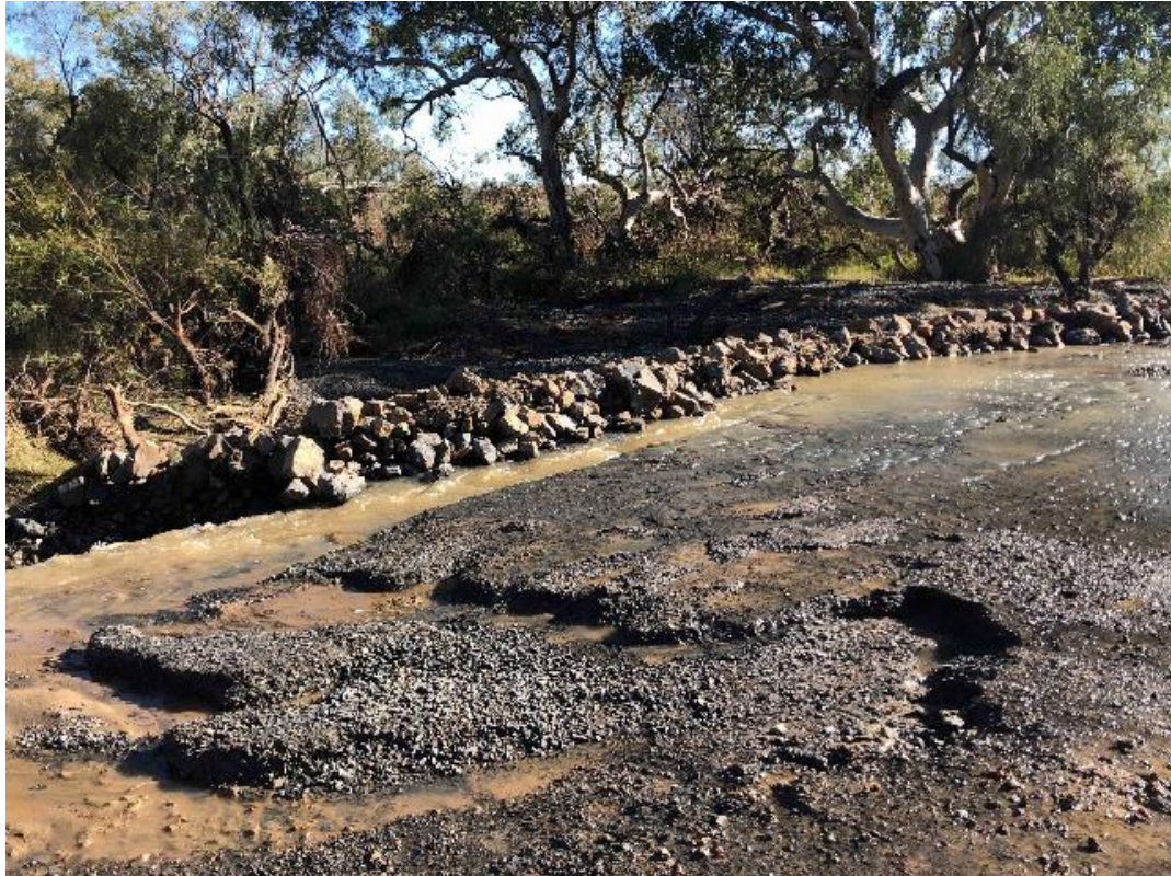
Plate 19 – Gurley Creek Bridge erosion to pad following rain event.
