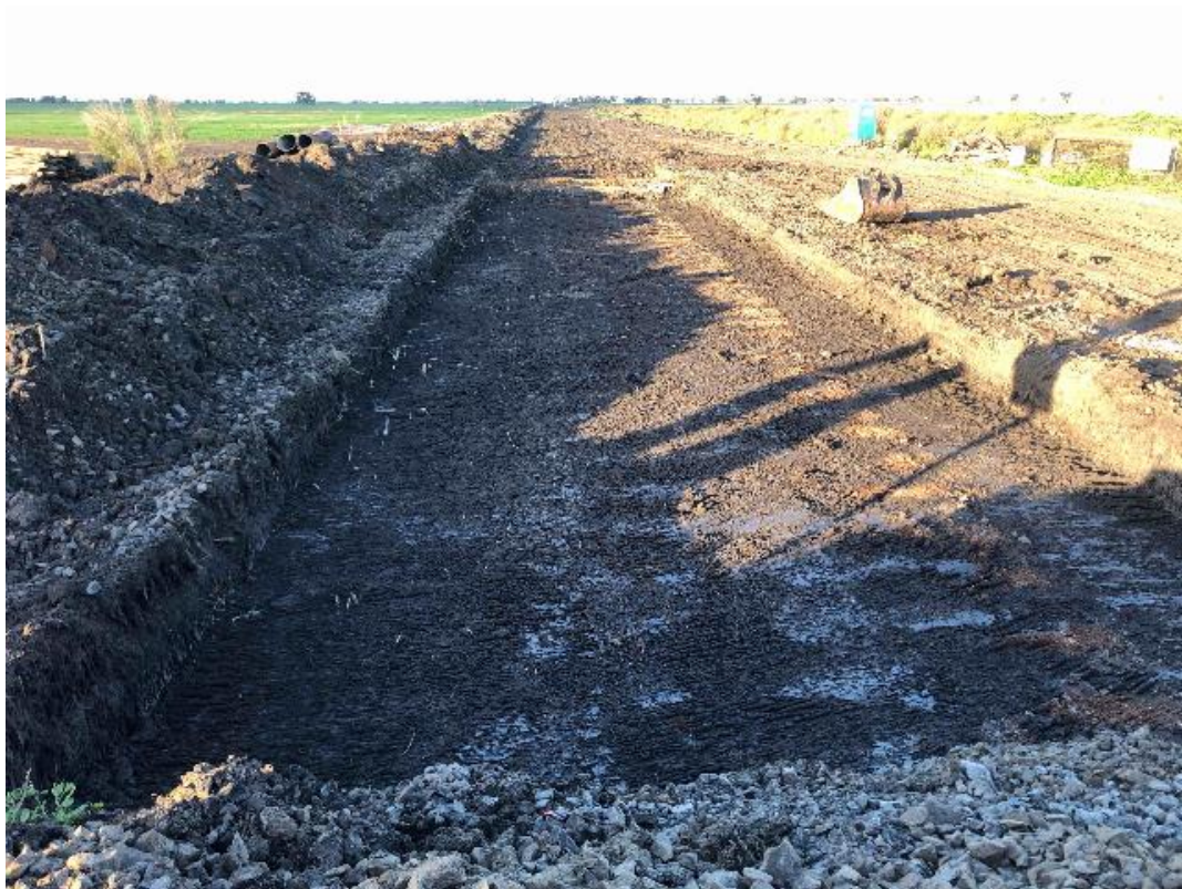
Plate 10 – Foundation and earthworks near Roydon Road level crossing.
