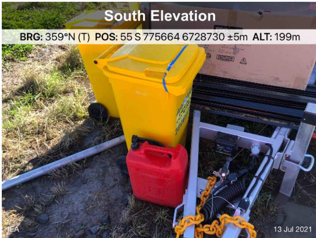
Plate 27 – Gurley Culverts Mill Rd – Fuel container not stored in bunded area adjacent ancillary facility.
