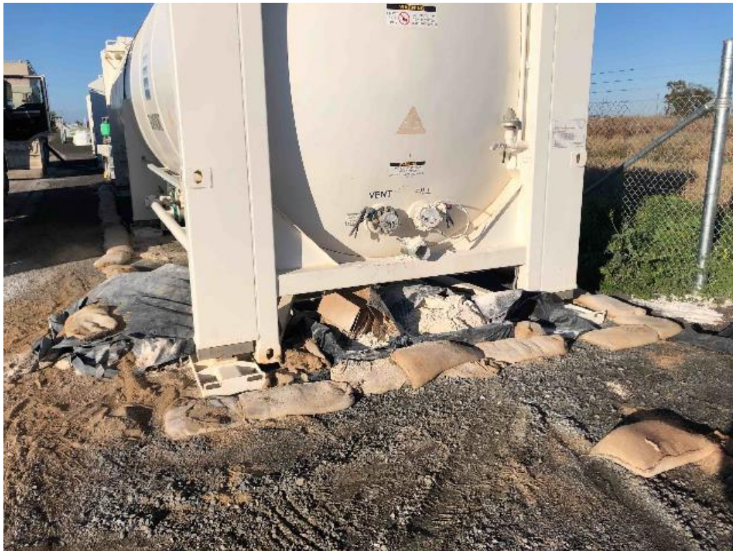
Plate 15 – PAD4 Lime storage tank with lime product located on ground surfaces
