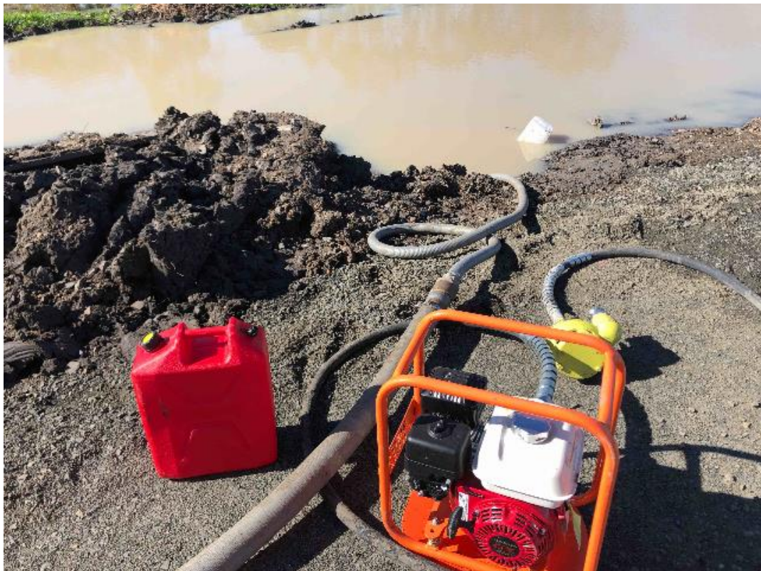
Plate 26 – Gurley Culverts Mill Rd fuel container adjacent pump in unbounded area.
