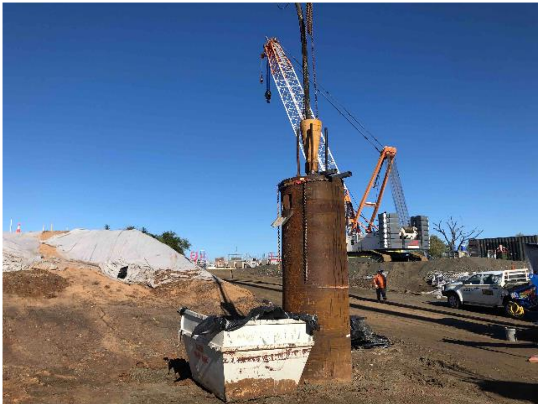
Plate 18 – Gurley Creek Bridge – Filling of pile with concrete with overflow bin installed at base
