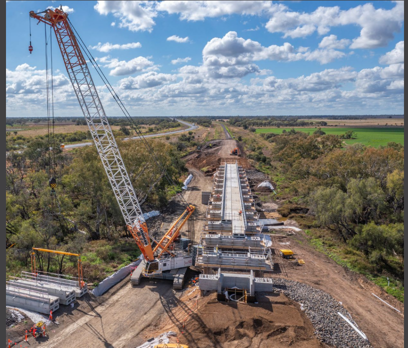
Construction work, Narrabri to North Star section – August 2021
