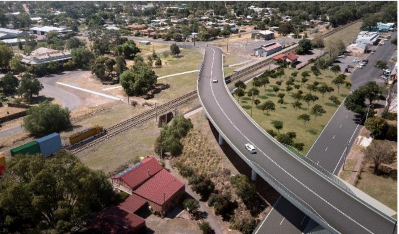
Created a corflute A0 poster to display in shop front window of vehicle overpass draft design option
