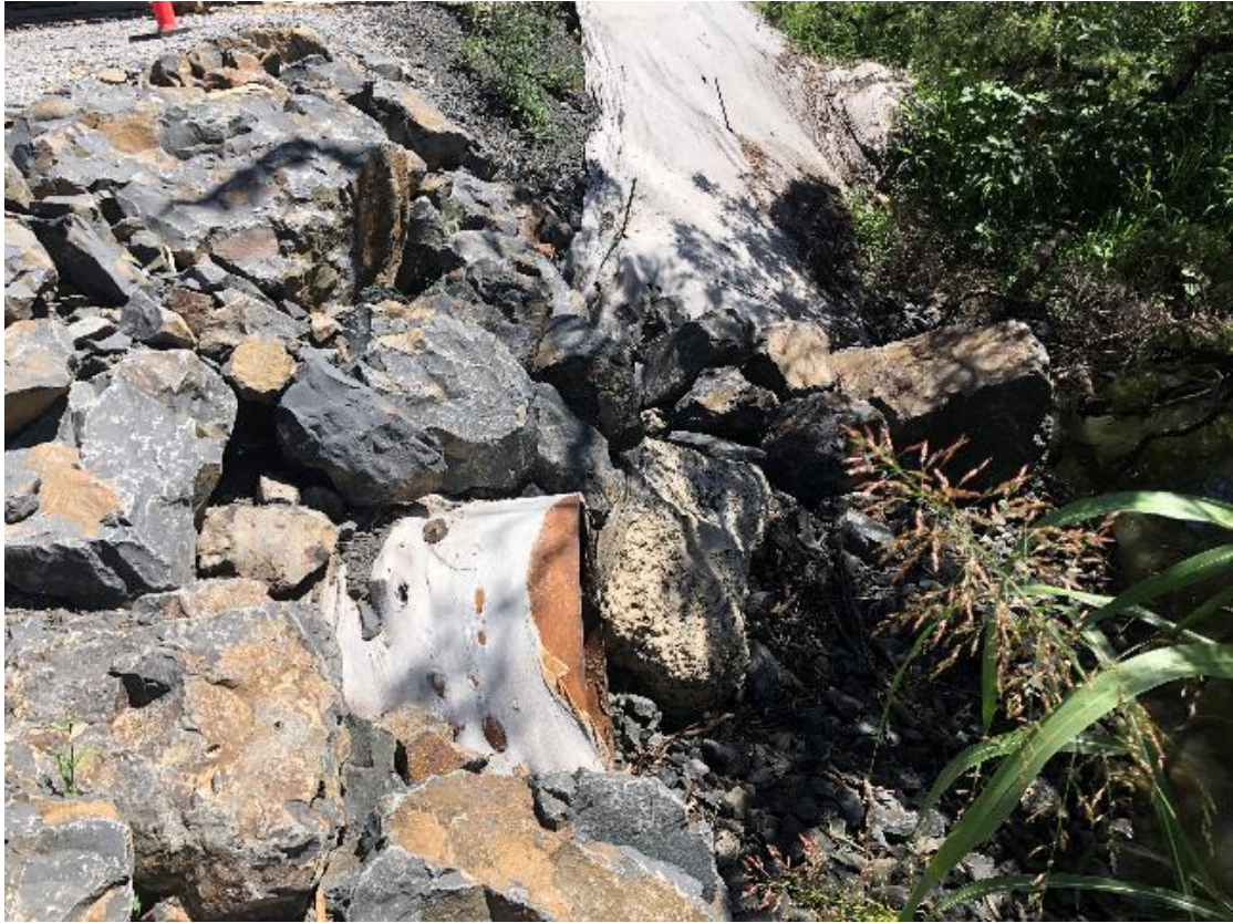
Plate 23 – Croppa Creek piling pad pipes
