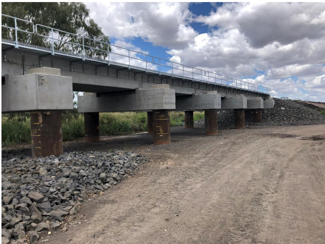
Plate 26 – Yallaroi Creek bridge completed
