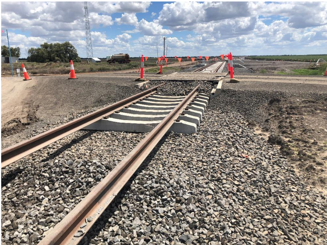
Plate 34 – Roydon Road Crossing and track installed
