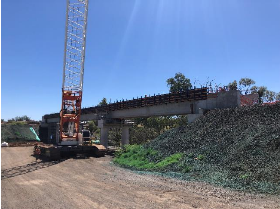
Plate 21 – Croppa Creek Bridge
