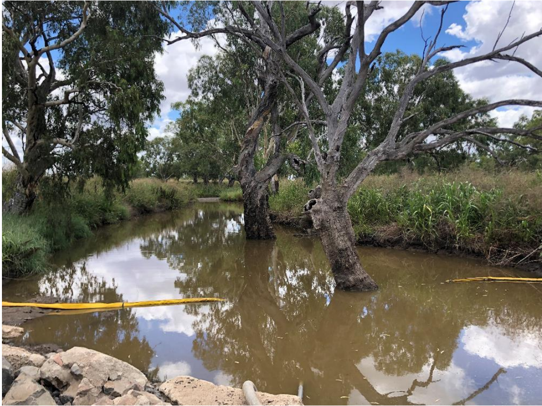
Plate 27 – Yallaroi Creek boom requiring repair
