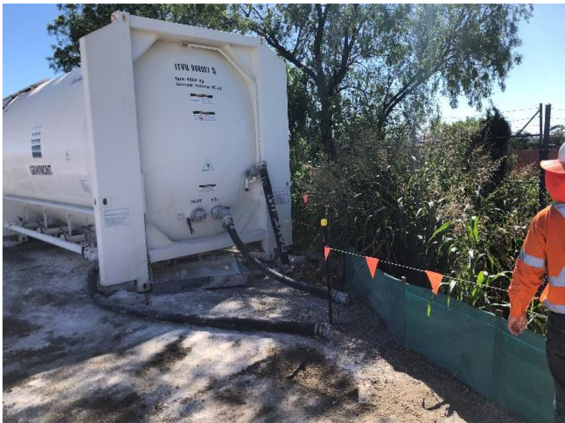
Plate 16 – Opportunity for improvement with sediment fencing installation - CroobleCrooble Laydown
