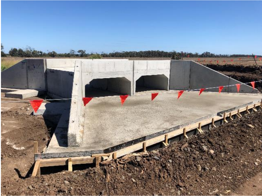
Plate 19 – Culverts installed along alignment – Chainage 736
