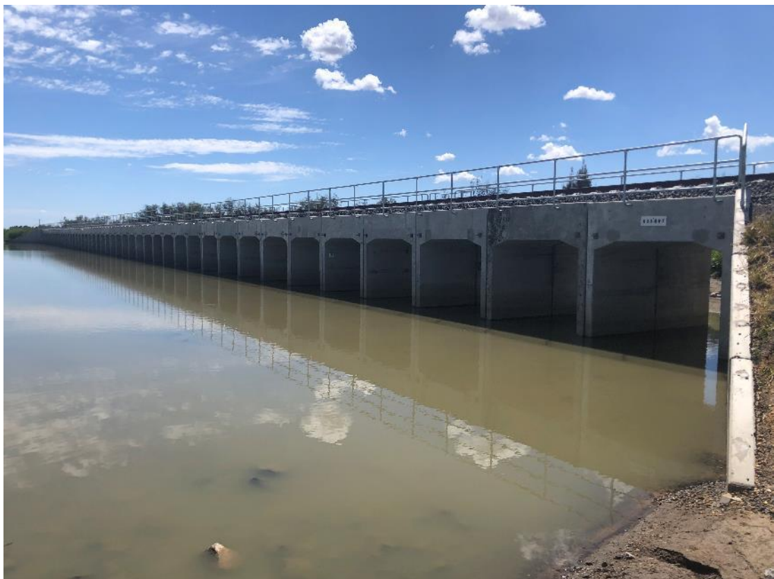
Plate 38 – Little Bumble Creek Culverts
