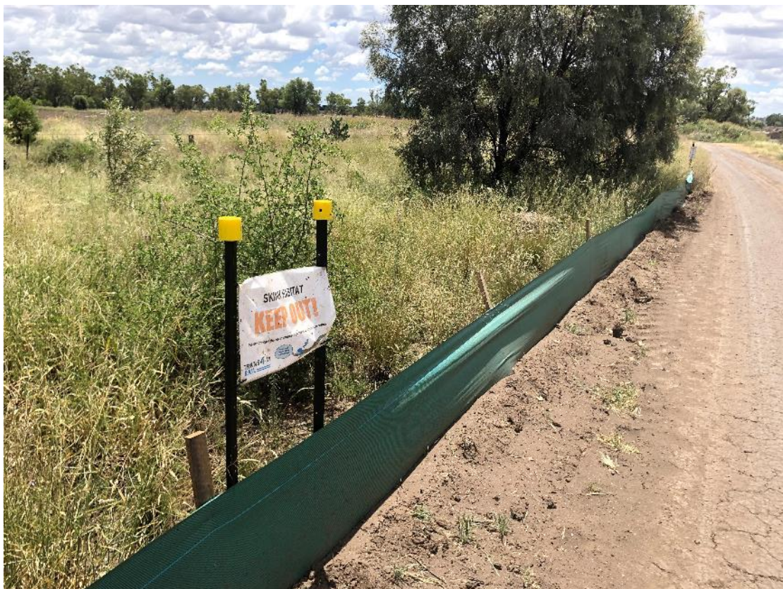
Plate 30 – Yallaroi Creek skink signage and sediment fencing in place
