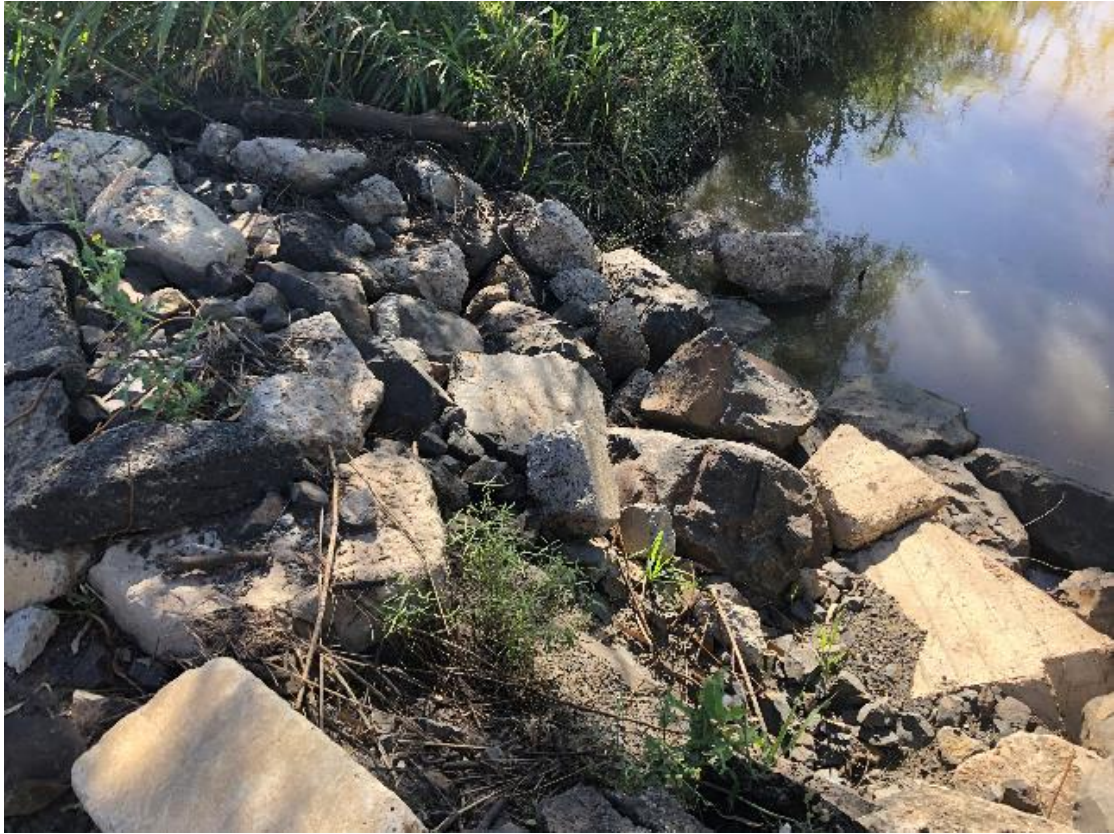
Plate 11 – Larger rock and materials used to stabilise Gil Gil Creek piling pad.
