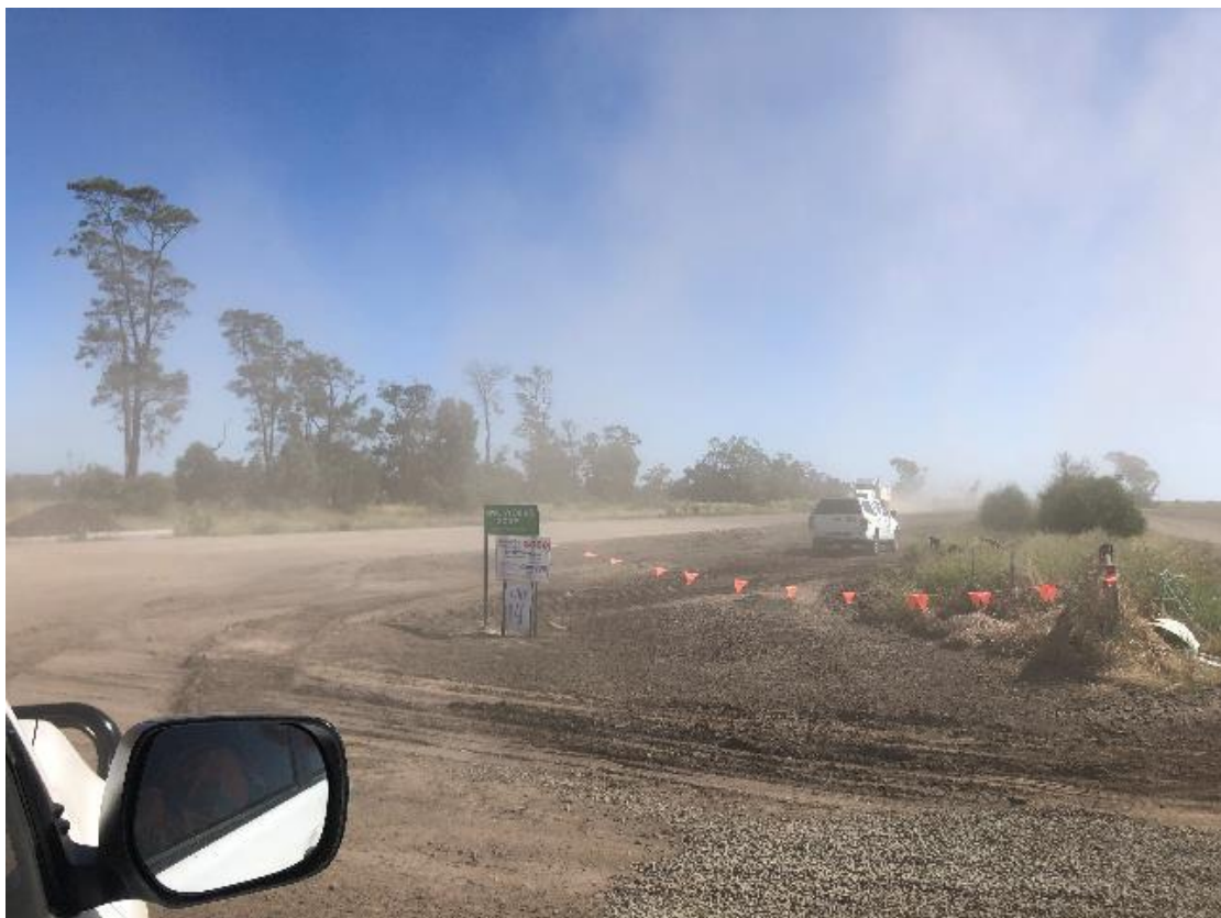
Plate 18 – Dust production caused by truck movements near Crooble Laydown
