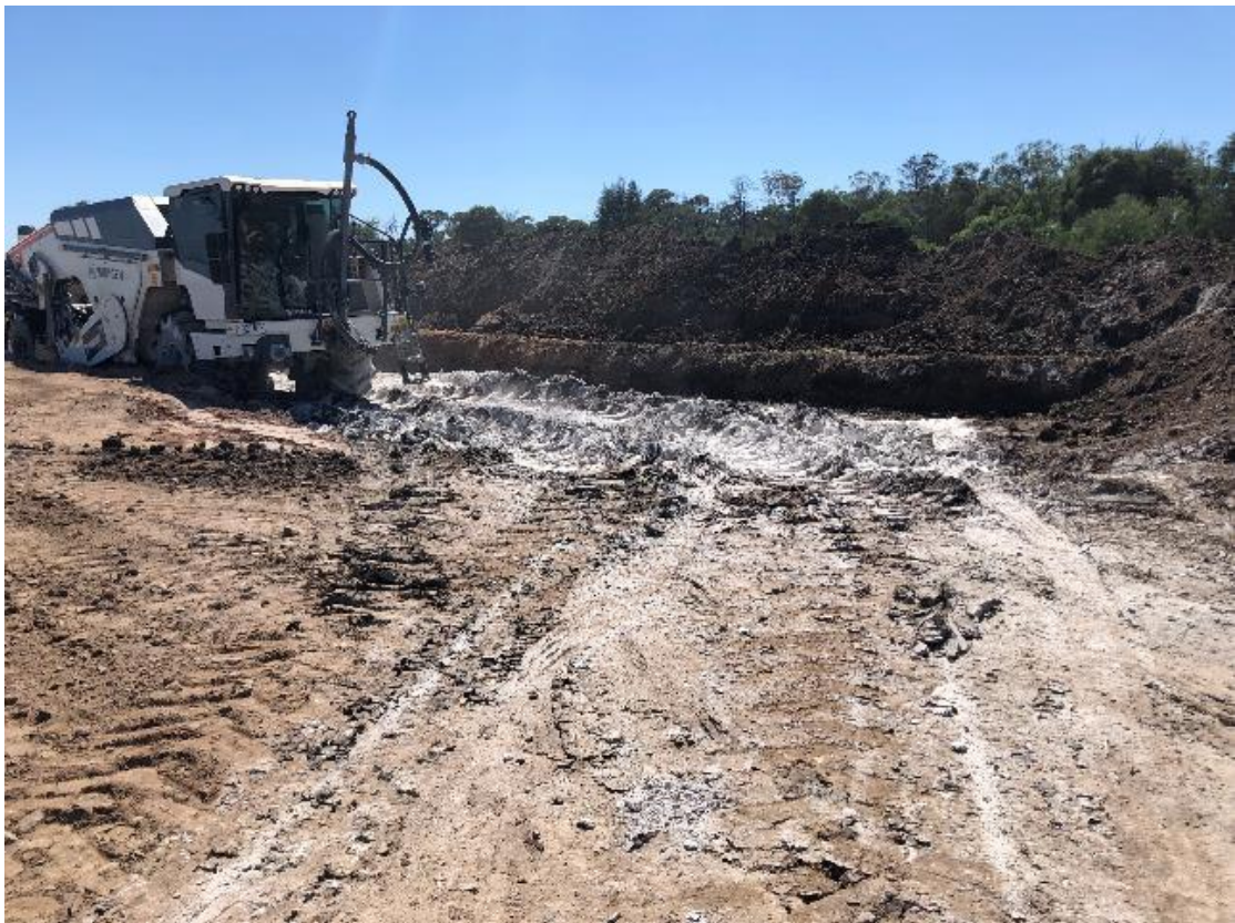
Plate 20 – Lime mixing along alignment
