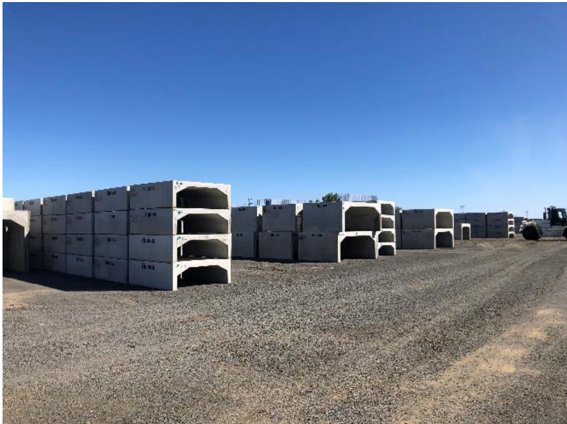
Plate 15 – CroobleCrooble Laydown – culvert sections
