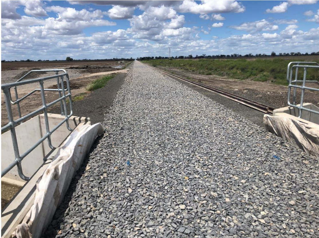
Plate 33 – Roydon Road Crossing top layer of ballast installed
