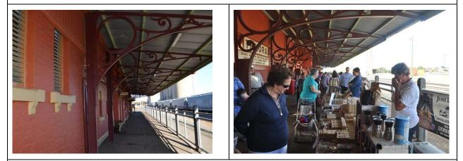
4. Two views of the disused platform at Temora Station. The station has been adaptively re-used as a community hub (see photograph to right), necessitating the unsympathetic additions of the platform edge barriers. Awning brackets are finished in yellow, similar to Cobar Station (source: NSW Government Architects [left], WikiCommons [right]).
