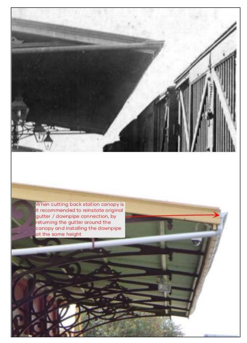
Figure 4-1: Down pipe connection as shown in 1925 (top image), versus 2021 (lower image).
