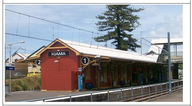
View of Kiama Station showing an alternative two-platform design necessitating a footbridge (Type 11). Ornate brackets are on both platform awnings with intrusive platform number labels (see image 9) (source: WikiCommons).
