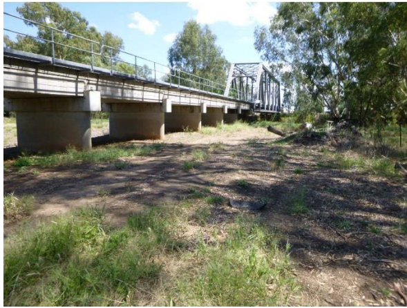
3. View of the approach spans facing north.
