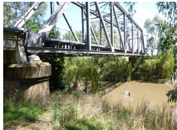
6. North view of the piers in relation to the bridge.
