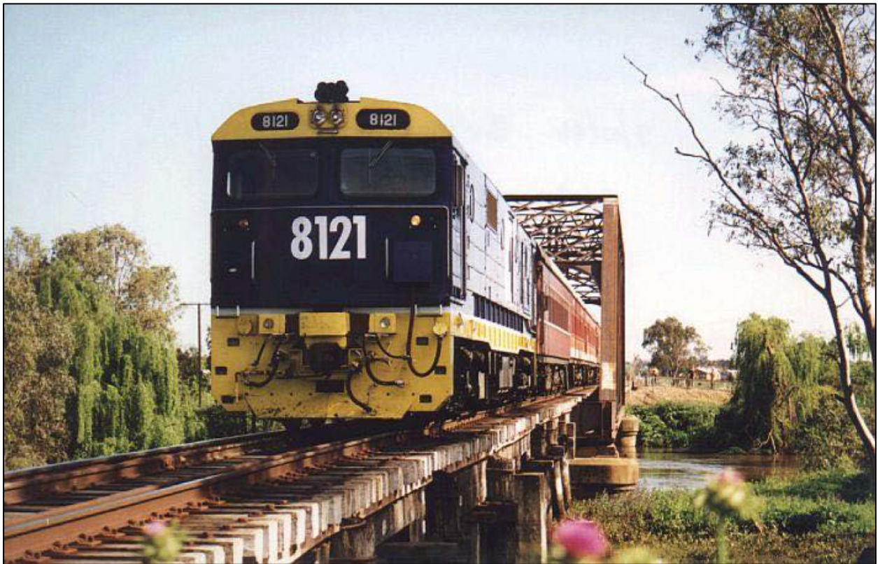
Figure 2-2: Image of the Lachlan River Bridge.
