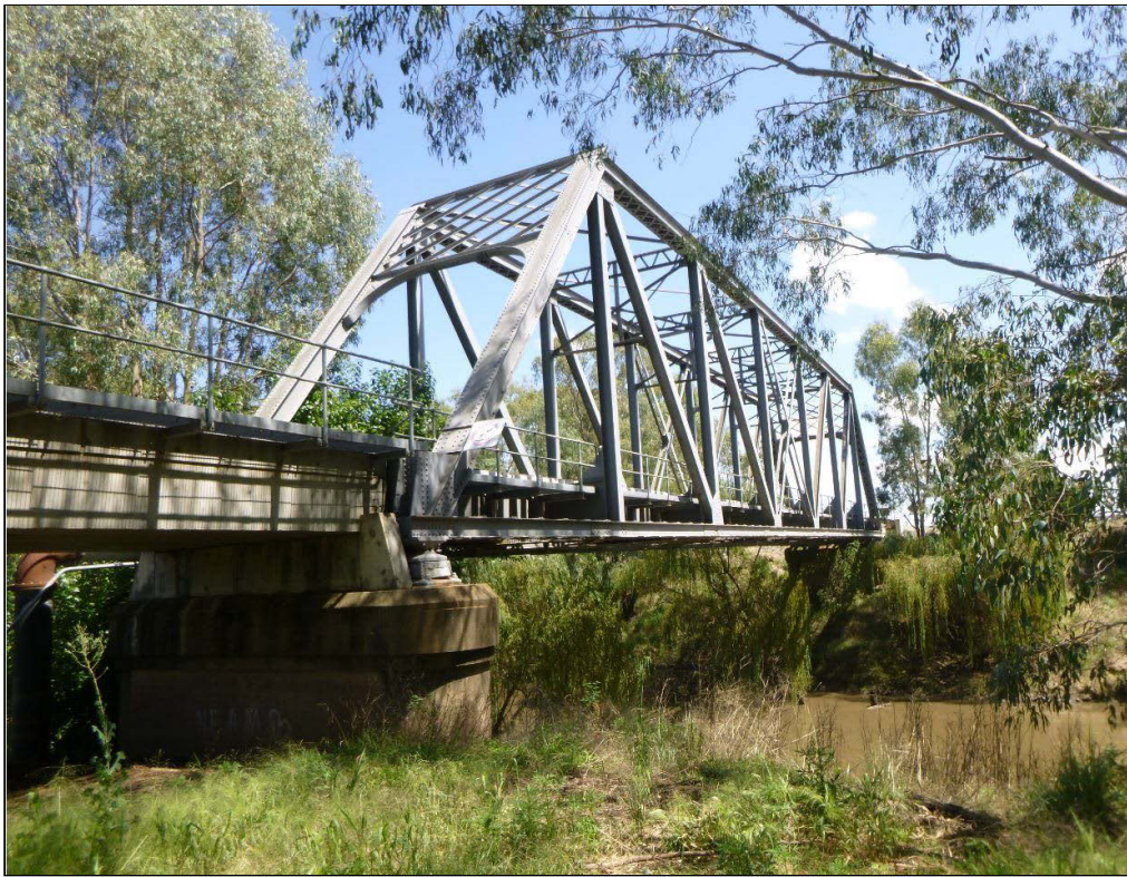
View of the Lachlan River Railway Bridge.
