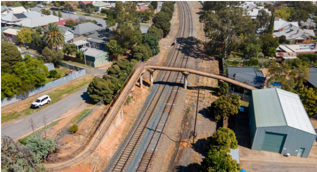
Existing Cassidy Parade pedestrian bridge
