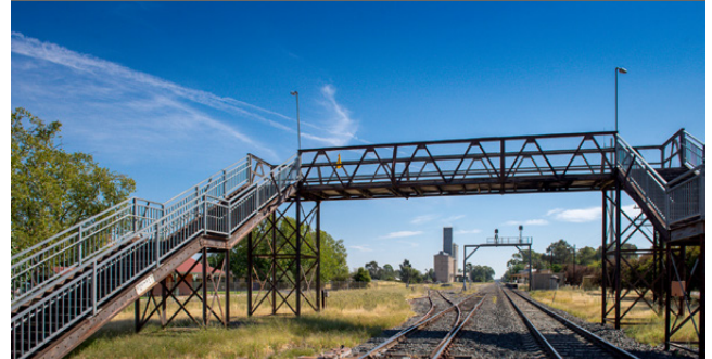
Culcairn pedestrian bridge
