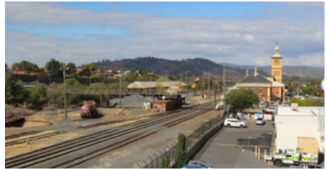
Albury Station pedestrian bridge – existing
