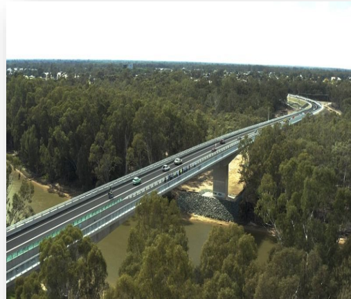
Echuca Moama bridge
