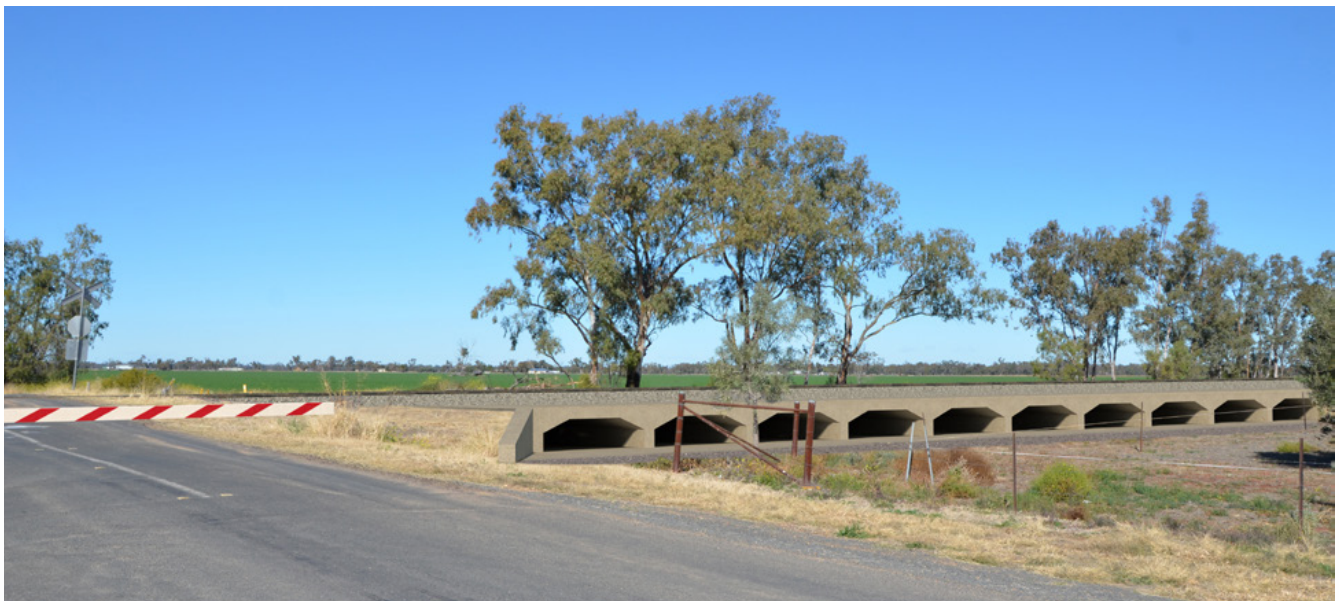
View from Gwydirfield Road level crossing – after
