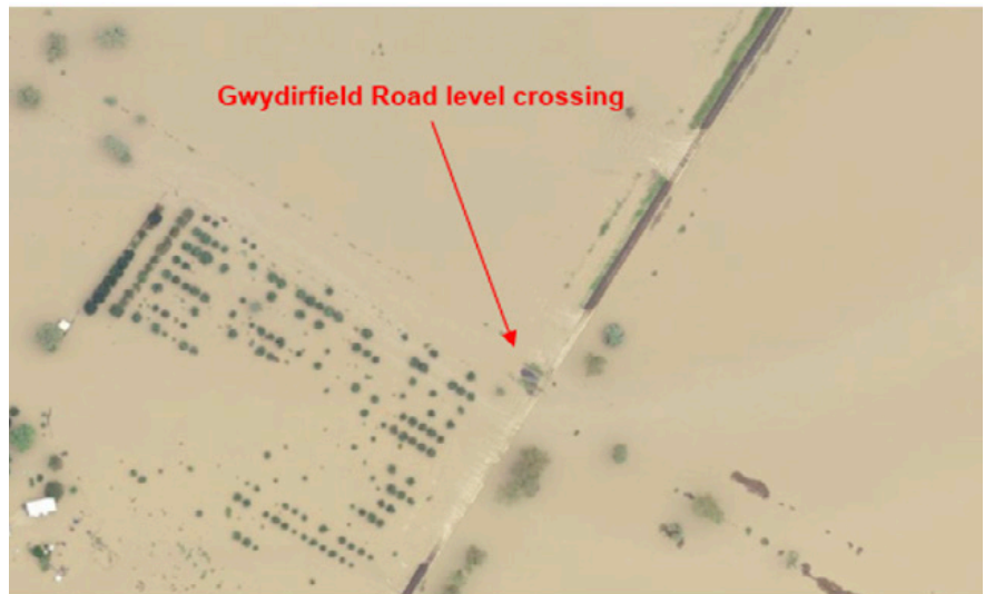
2012 flood showing washouts of the rail line
