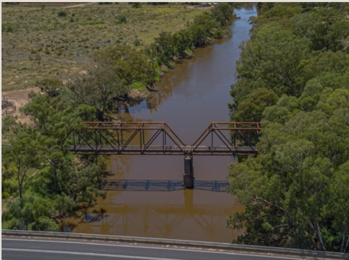
Gwydir River Bridge
