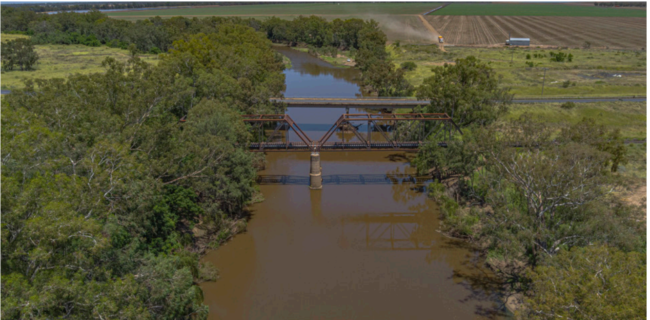
Gwydir River Bridge
