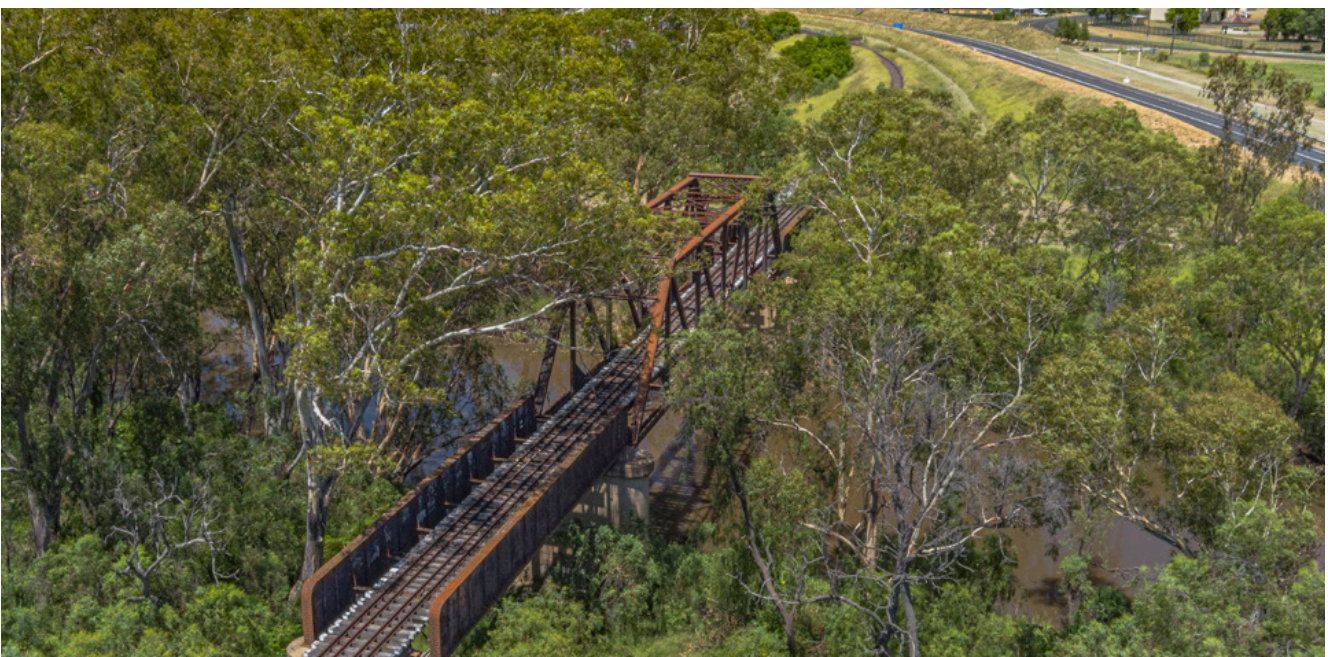
Mehi River Bridge
