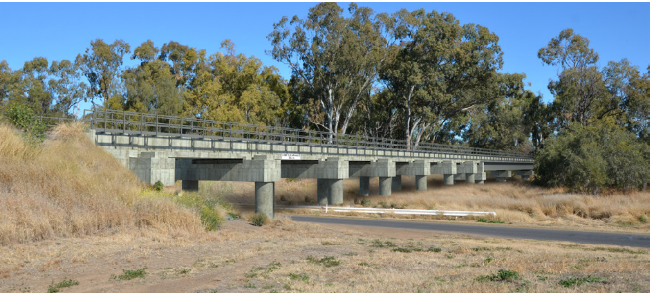
Mehi River and Gwydirfield Road crossing – after
