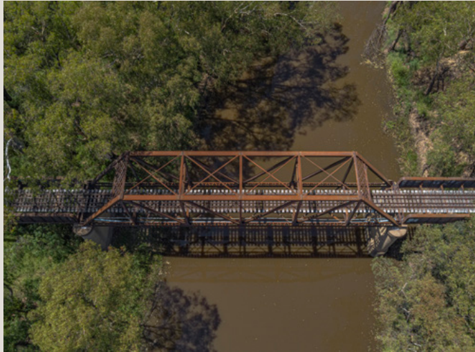
Mehi River Bridge
