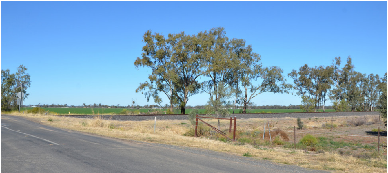
View from Gwydirfield Road level crossing – before
