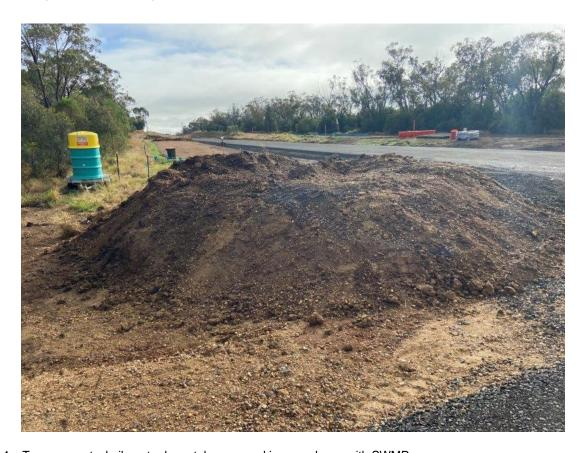
Plate 4- Temporary stockpile not adequately managed in accordance with SWMP
