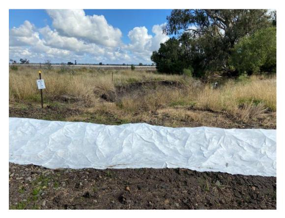
Plate 22 – Sediment control structures within CIZ along with signposting at Gate 7  $\,$
