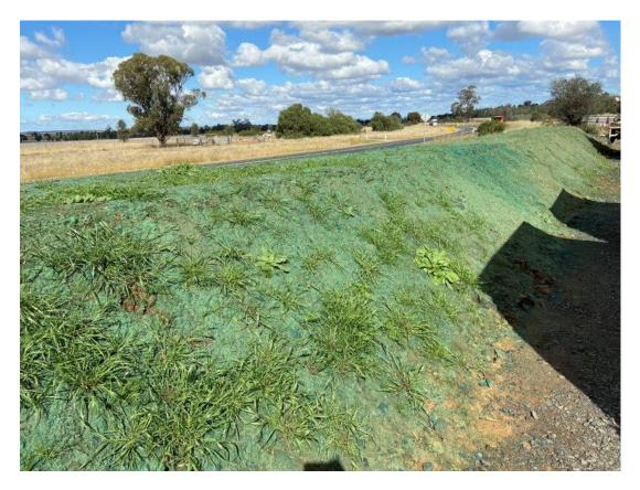
Plate 24 – Spray grass applied to batter
