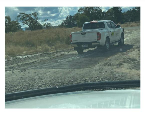
Plate 23 – Rumble grid utilised at Gate 7 MAF
