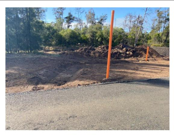
Plate 9 - Temporary stockpile not adequately managed in accordance with SWMP along alignment CH621
