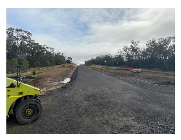
Plate 3 – Subgrade installed in alignment
