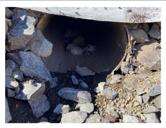
Plate 27 – Bobbiwa Bridge minor material located within pipes
