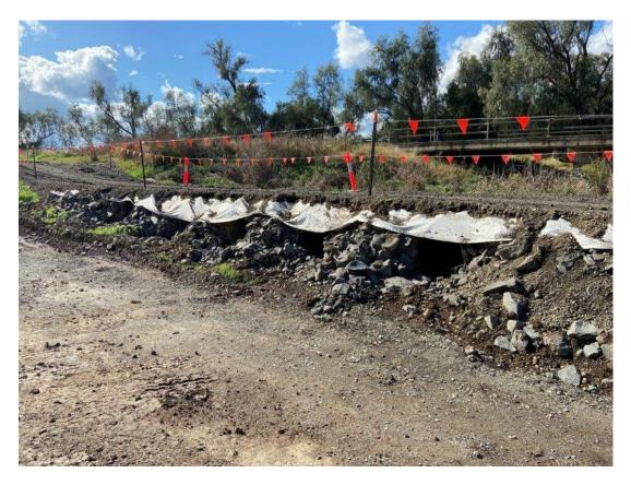
Plate 26 – Bobbiwa Bridge evidence of erosion of rock protection
