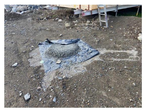
Plate 32 - 10 Mile Creek concrete spillage on piling pad
