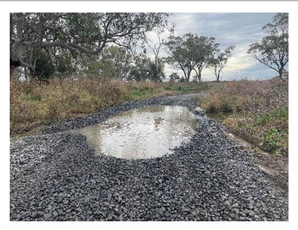
Plate 37 – PAD 2 Gurley Bridge causeway with indications of sediment migration and erosion downstream
