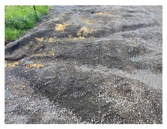
Plate 30 – 10 Mile Creek Bridge evidence of pad erosion
