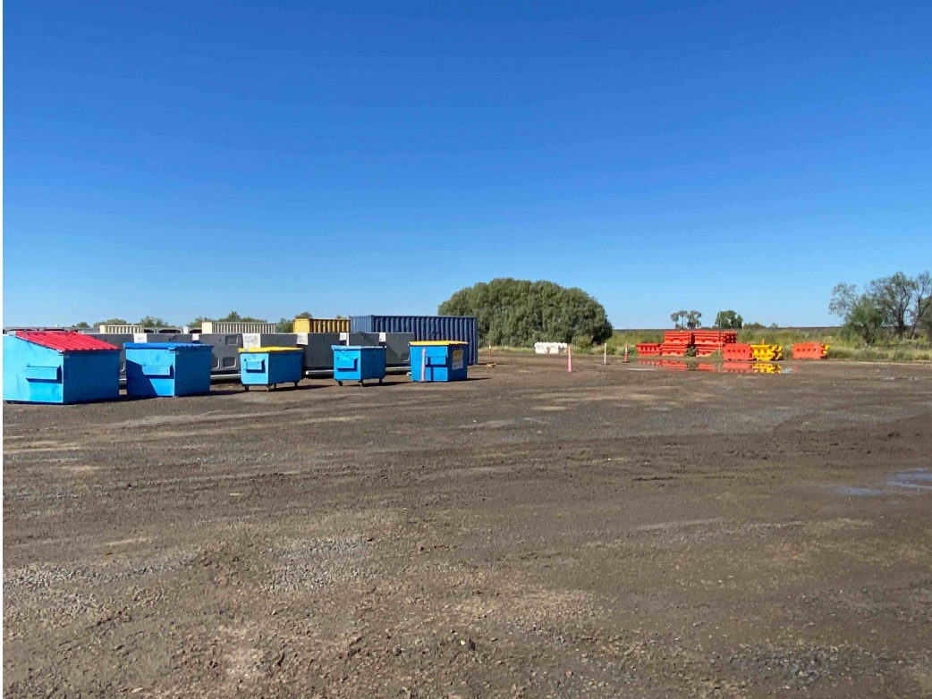
Plate 5 – Pad 2 stockpile and materials laydown area
