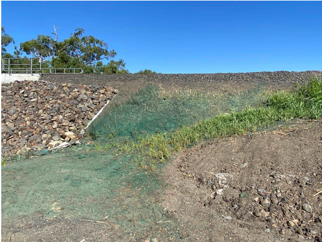
Plate 21 – Hydromulch applied at batter adjacent to Gil Gil Creek
