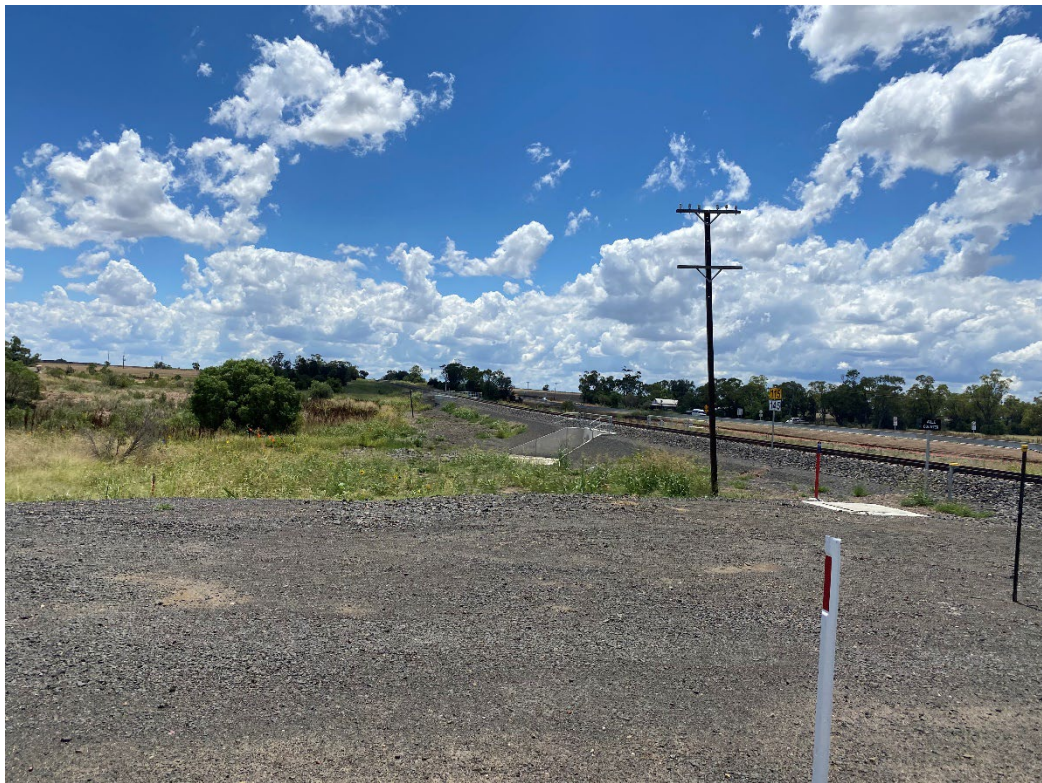
Plate 12 – Millie Road LX looking north
