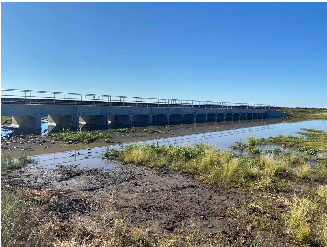
Plate 2 – Culverts over Clarks Creek
