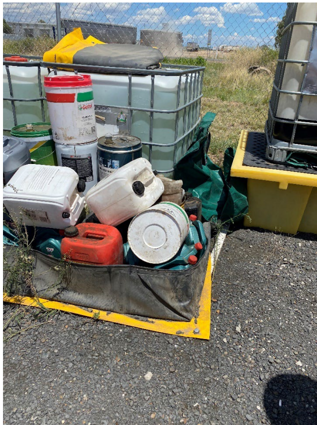
Plate 14 – Overfilled bund with collapsed sides at Pad 4
