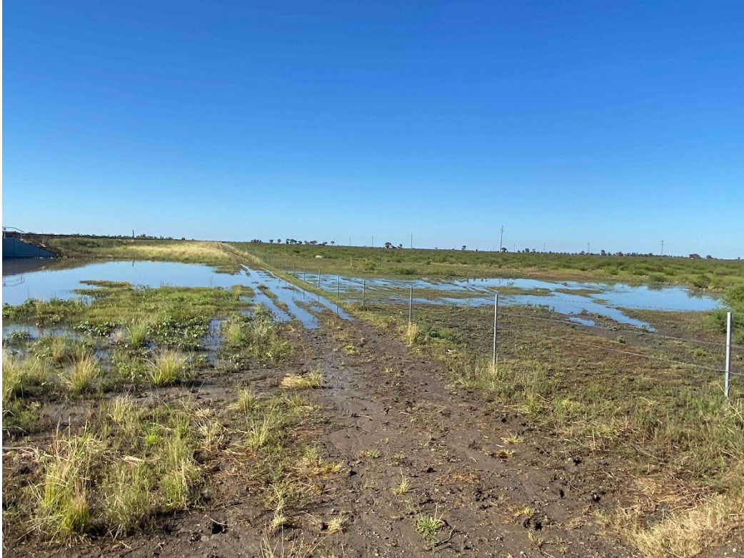
Plate 3 – Overflow from Clarks Creek, flooding access road
