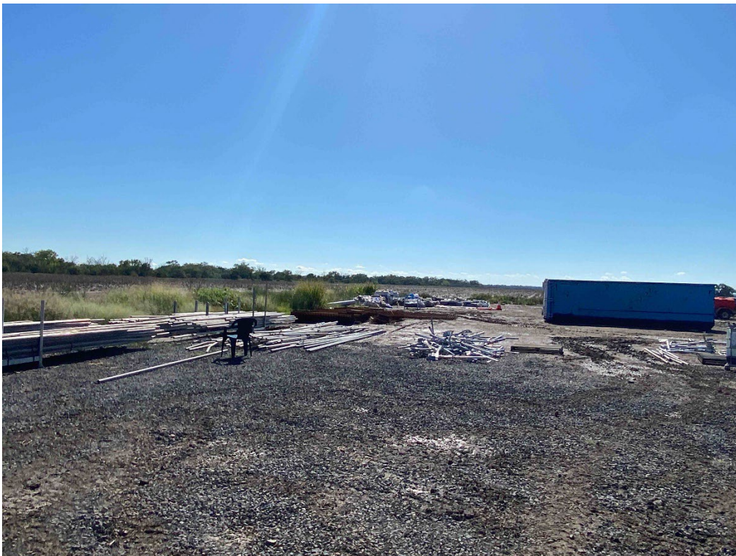
Plate 6 – Stockpile and laydown area at Pad 2
