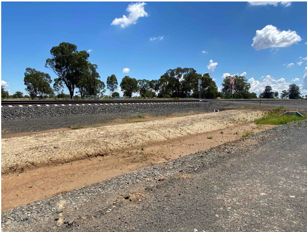
Plate 8 – Drainage channels at Gate 2
