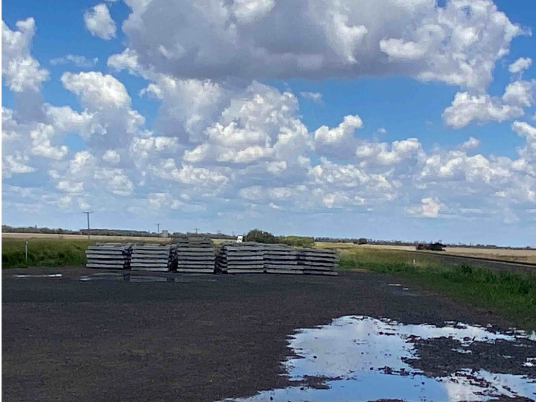
Plate 11 – Clump Road laydown area
