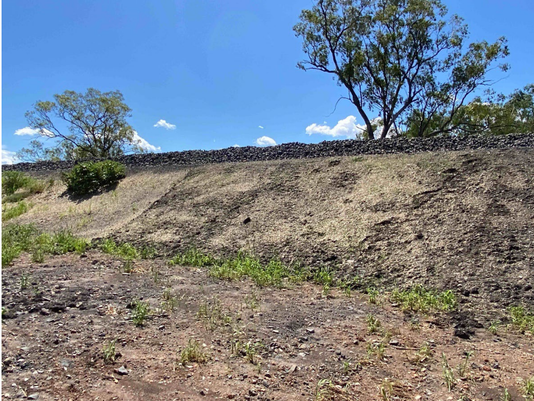
Plate 25 – Embankment batters along alignment near Croppa Creek tributary
