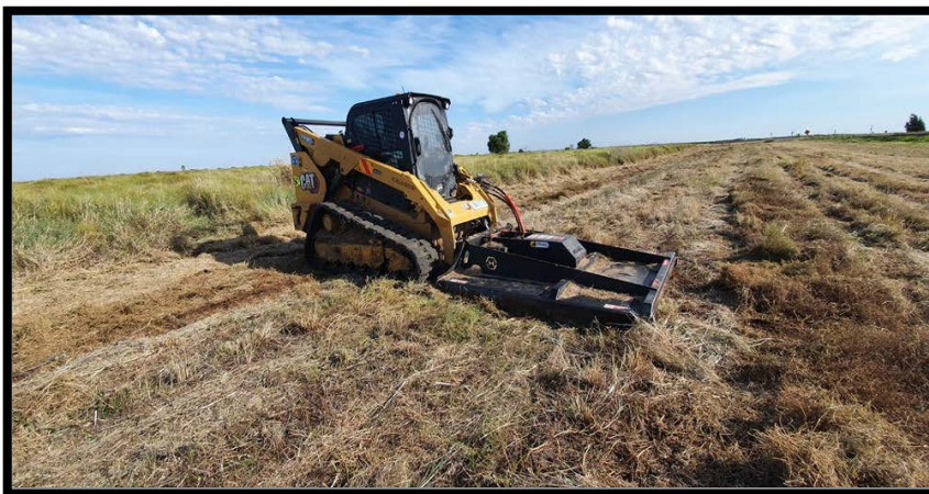
Figure 5-3: Slashing on vegetation prior to stripping at N2NS SP1.
