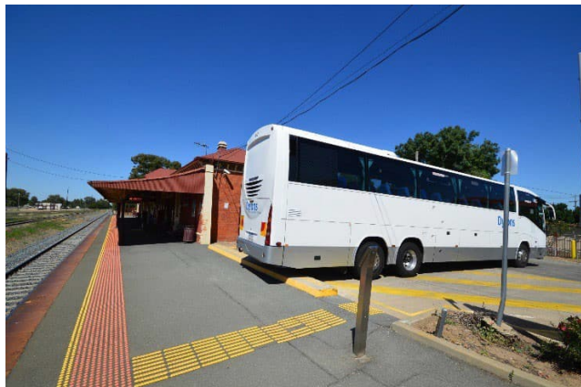
A coach attempting a three-point-turn maneuver south of the station. The lack of sufficient space for bus circulation results in a dangerous impediment upon the station's northern platform. As a result, commuters are put at risk despite visual and tactile warnings.
