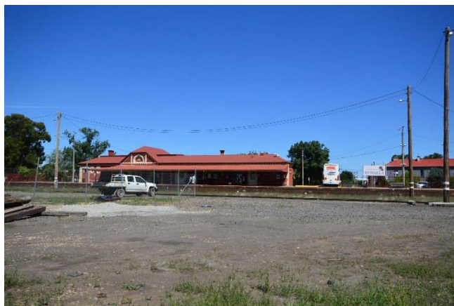
View south towards the station from the northern land expanse. The expanse comprises of disorganized, unused, or wasted rail assets, which are observed upon arrival to Benalla.
