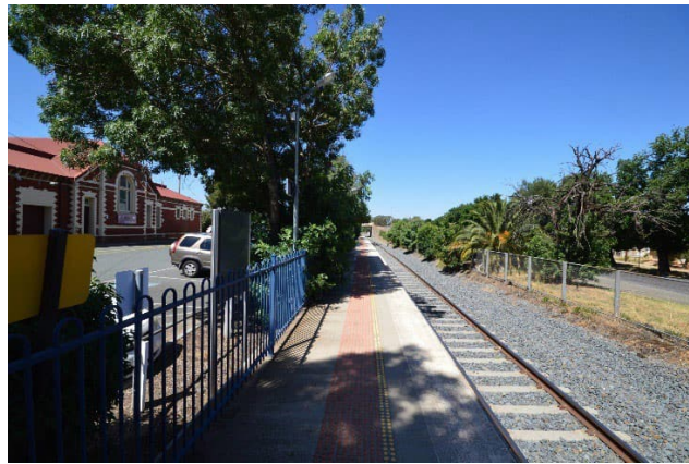
View east observing the existing platform south of the station. The platform's width has been cited as a safety concern due to poor visibility because of its width.
