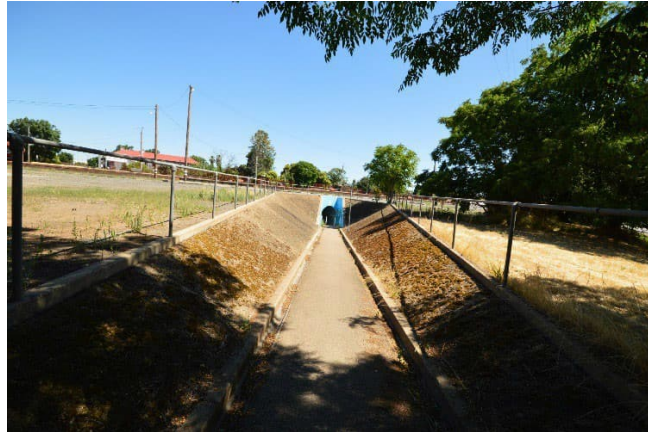
Ramp and associated stabilised embankments upon descent into the pedestrian underpass from Railway Place.
