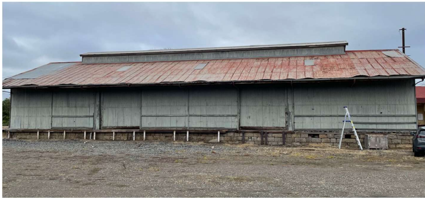
Images 3-14 – General condition of roof sheeting, view from Down Side
