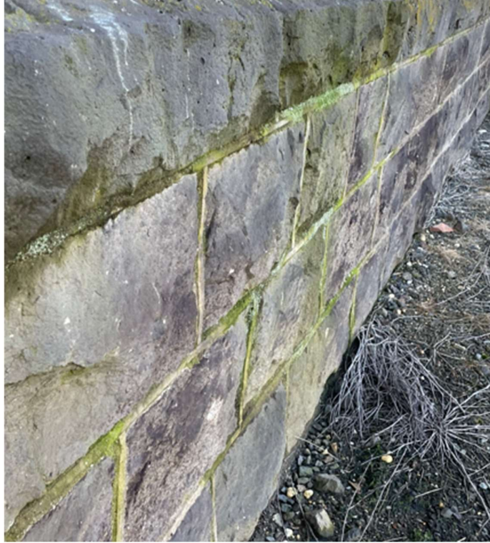
Image 3-35 – Bluestone upstand generally in good condition
