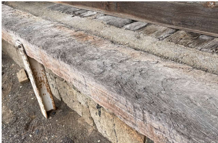
Image 3-30 – Typical condition of timber beams
