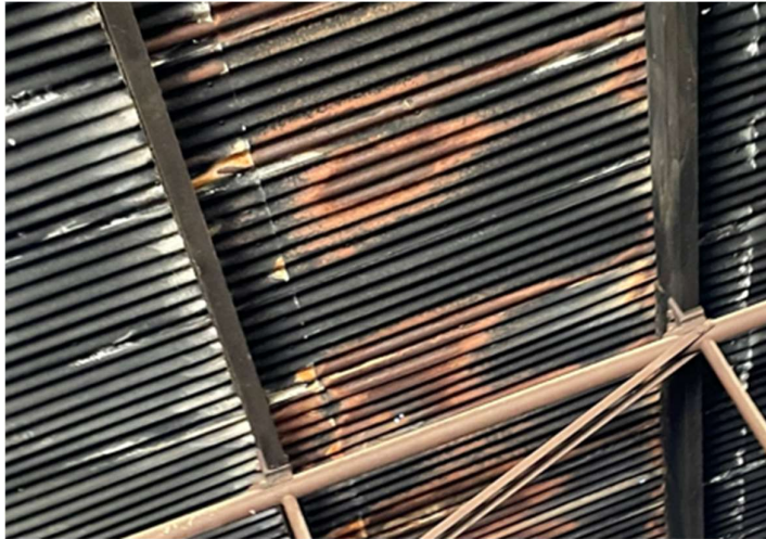
Image 3-23 – Typical condition of purlins
