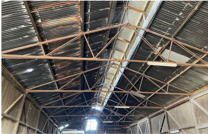
Images 3-10 – Steel roof trusses, generally in good condition
