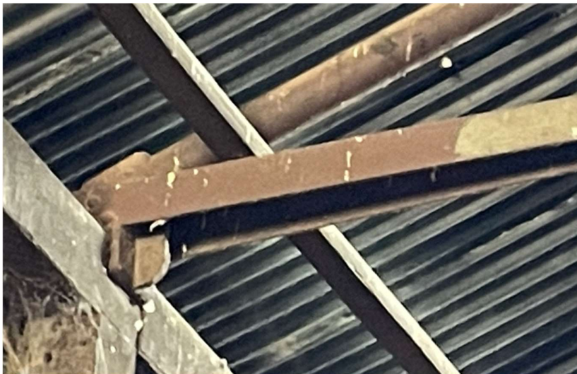
Images 3-13 – Steel roof truss connection to timber beam
