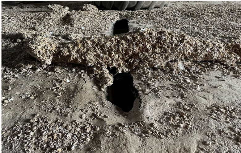
Image 3-40 – Failed timber deck poses a serious risk of injury
