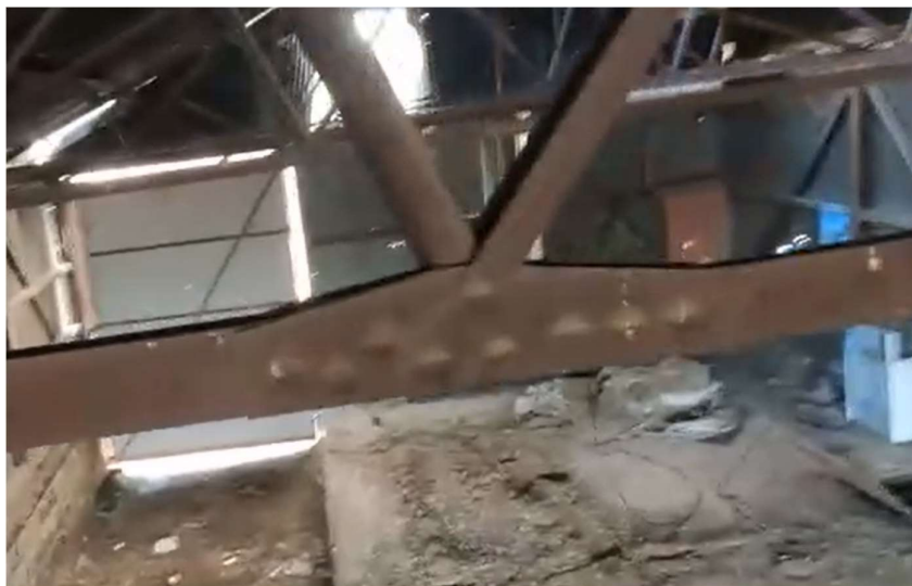
Images 3-11 – Steel roof truss connection (image taken via Go-Pro on pole)
