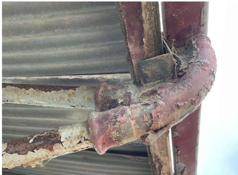
Images 3-22 – Typical condition of fascia supports at connection to gutter
