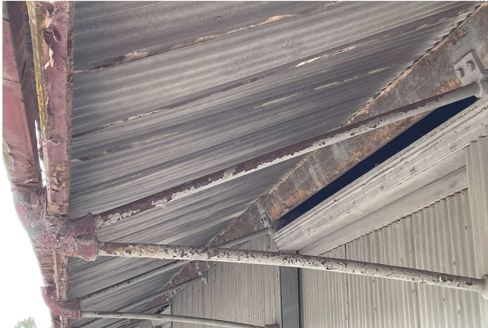
Images 3-21 – Typical condition of fascia supports (strut and ties)
