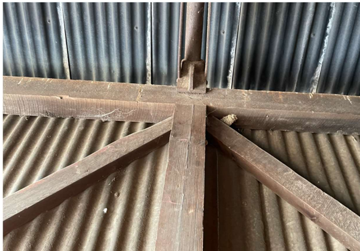
Image 3-31 – Typical condition of timber bracing
