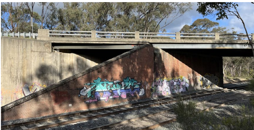
The design of the new bridge will include removal of the middle pier.
